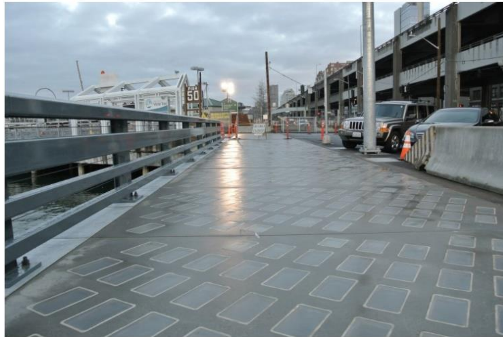
A segment of the new Seattle seawall. The sidewalk's light-penetrating glass panels let light through to the water below to encourage young salmon to migrate along the engineered shoreline. SDOT/Flickr
