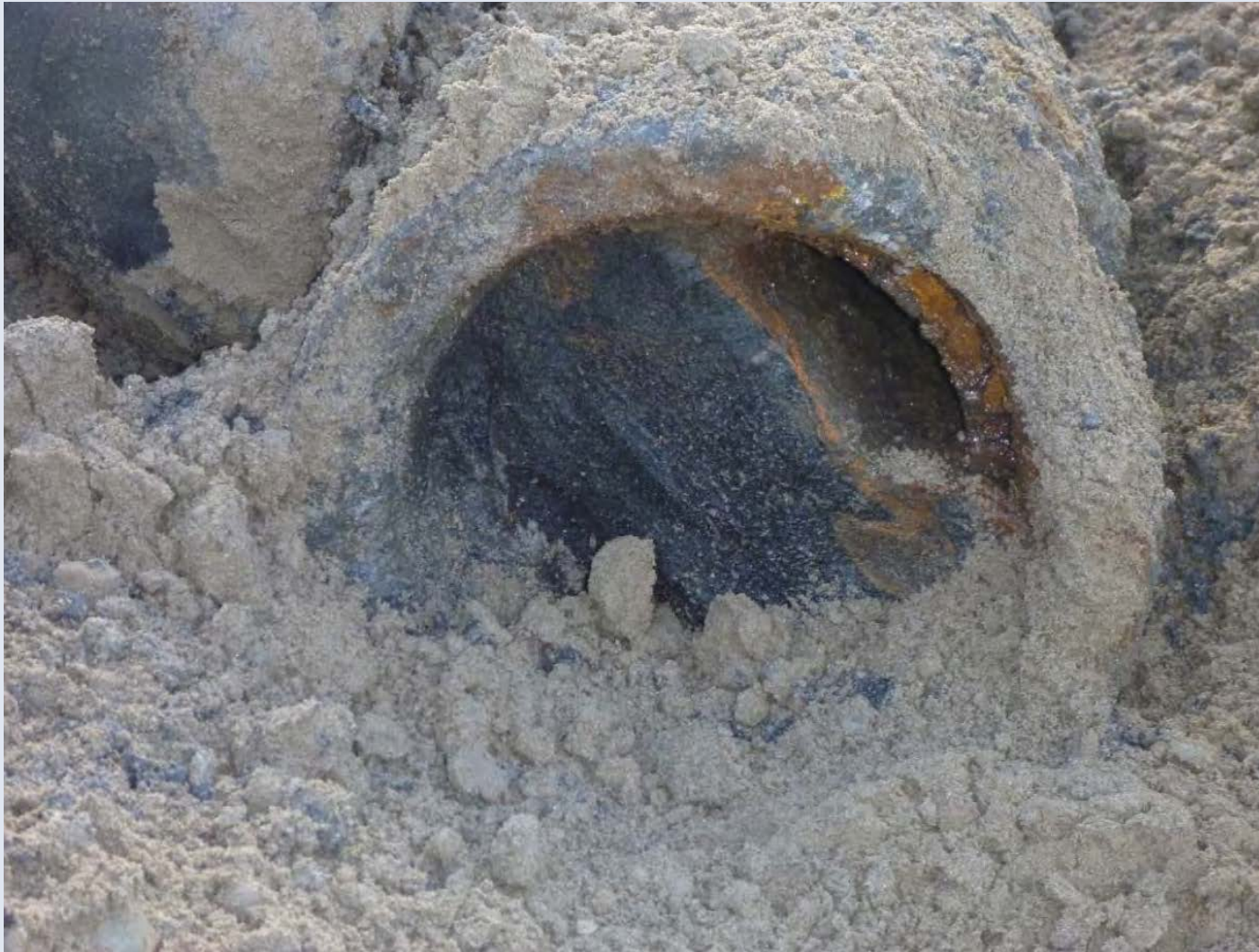
Sandblast Grit Encountered in Former Storm Drain Pipe
