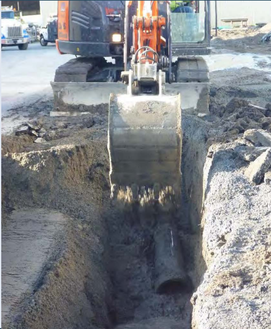
Removal of Storm Drain Pipe
